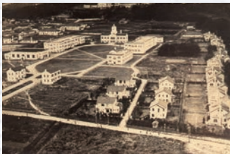
Aerial View : Uegahara Campus After Completion
